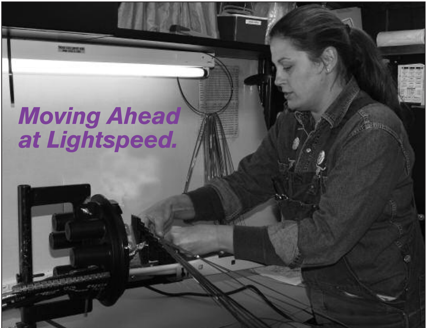
Jeanne Lindenmuth of the New Lennox garage works on fiber splicing in Lockport.
